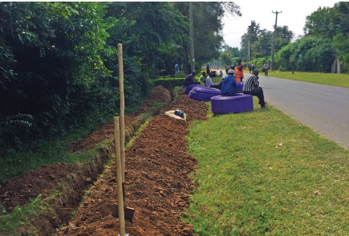
Fibre optic cables being laid across Kisumu City by Liquid Telecom.
